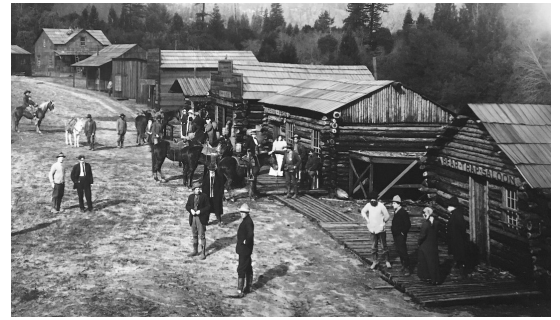
CMPC built this entire western town set in the Santa Cruz Mountains to film Salomy Jane Source: MHM
